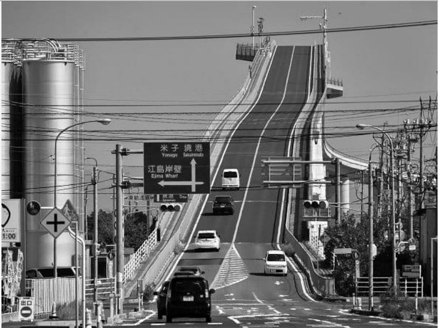
The 'Roller coaster' bridge linking the Japanese cities of Matsue and Sakaiminato was constructed like this in order to enable large ships to pass beneath on Lake Nakamui
