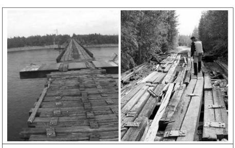
The rotting Vitim River Bridge is in Siberia. Once a rail bridge, the structure has long since fallen into disrepair, its wooden platform decaying and its dangers all too obvious. The bridge measures 1900 feet long and just six feet across and is not much wider than most modern motor vehicles. With no rail or barrier, there's little to stop drivers plunging into the freezing waters below.
