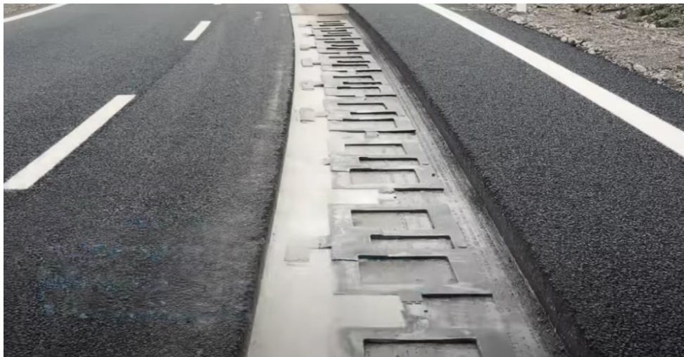
Under the asphalt, the DWPT system has a series of inductive charging coils Stellantis
